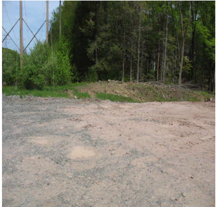
Old Farms Rd: Stockpile upgradient from wetlands has been fully removed.
