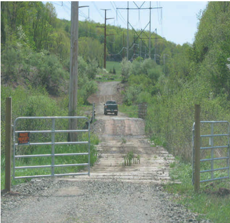
Durham Rd: Contractor measuring the length of the access road has driven through the flooded timber mats. Keep off mats when flooded if feasible.
