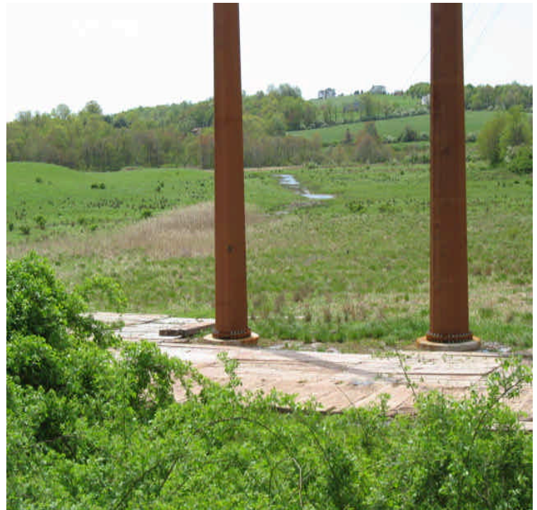
Tamarack Swamp Rd: View of timber mat staging area within wetland
