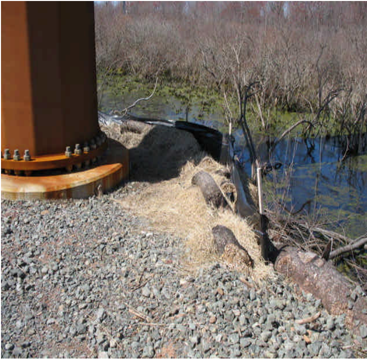
Tamarack Swamp: Controls remain at the edge of the pad to stabilize soils adjacent to the standing water.
