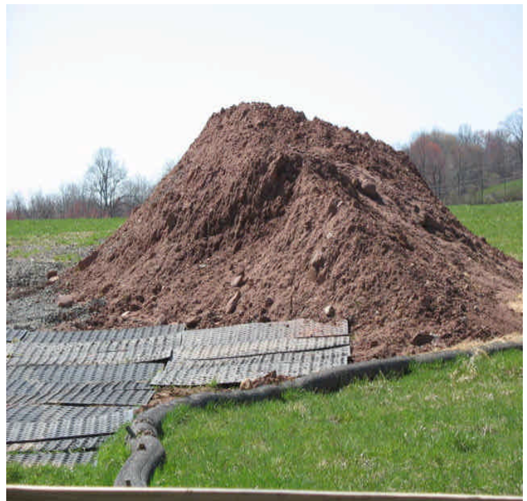
Tamarack Swamp Rd.: Stockpile located east of the roadway is not fully contained with controls. Add controls or stabilize or remove the stockpile.
