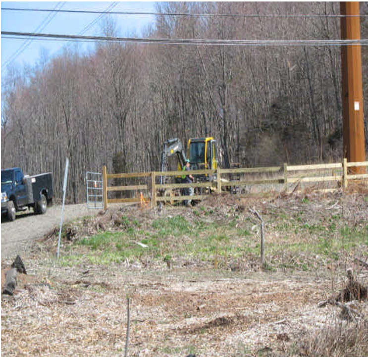
Durham Rd: Fence installation was underway north of Durham Rd.
