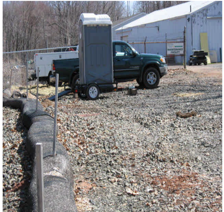
Harrison Rd: Sanitary facility located above a steep bank to a stream. The resource area appears to be greater than 100 feet away but relocate from the top of slope if feasible, in case of a spill.
