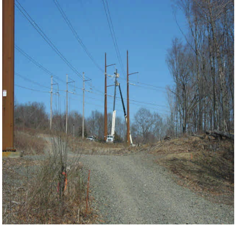
Durham Rd: Line work was underway.
