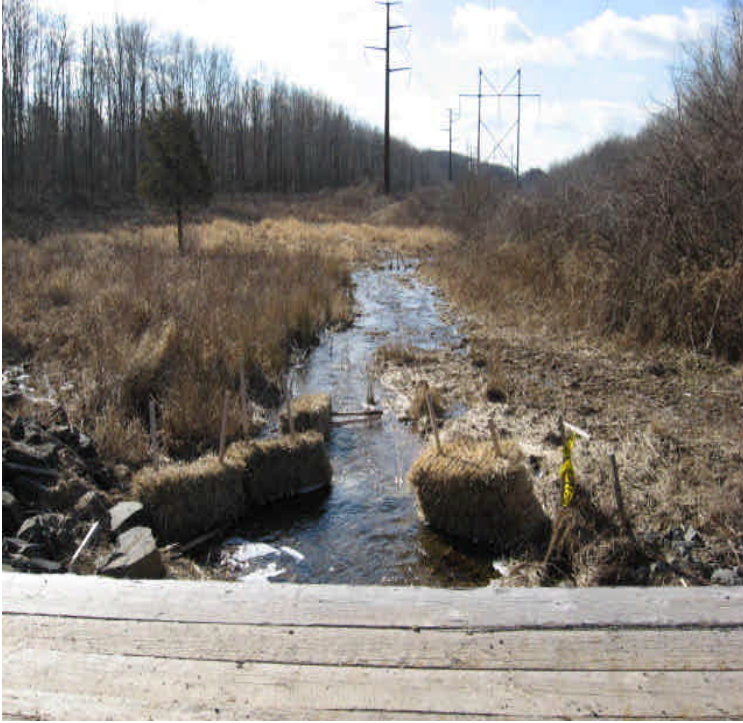
Carpenter Lane: Haybales have been knocked over at the wetland outlet due to high flow. ATVs continue to damage controls and leave tracks in wetlands.
