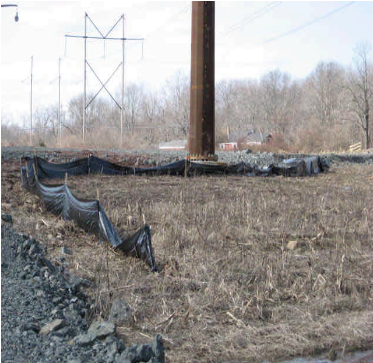
Tamarack Swamp Rd.: Silt fence has been repaired.
