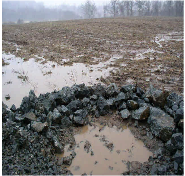
Tamarack Swamp Rd (east): Turbid run-off was observed flowing from the exposed farm fields and into the project's existing controls. However, the turbid water is not associated with the project.
