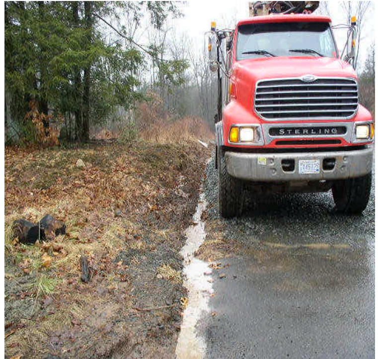
Old Farms Rd: Turbid water noted flowing down the drainage channel at the saturated driveway crossing and onto the roadway. Evaluate alternatives such as haybale check dams.
