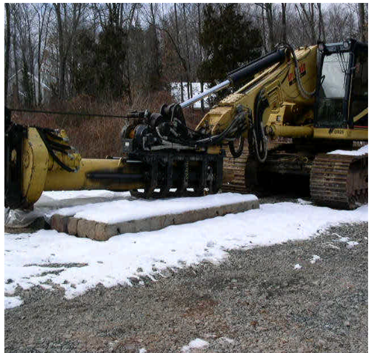
Old Farms Rd: Leaking equipment has a plastic tarp to contain drips. However, fluid is still washing onto the ground off the tarp. Leak should be repaired as soon as possible.
