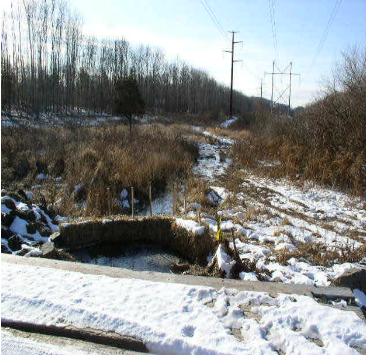
Carpenter Lane: Haybales remain at the wetland outlet. ATVs continue to damage controls and leave tracks in wetlands.
