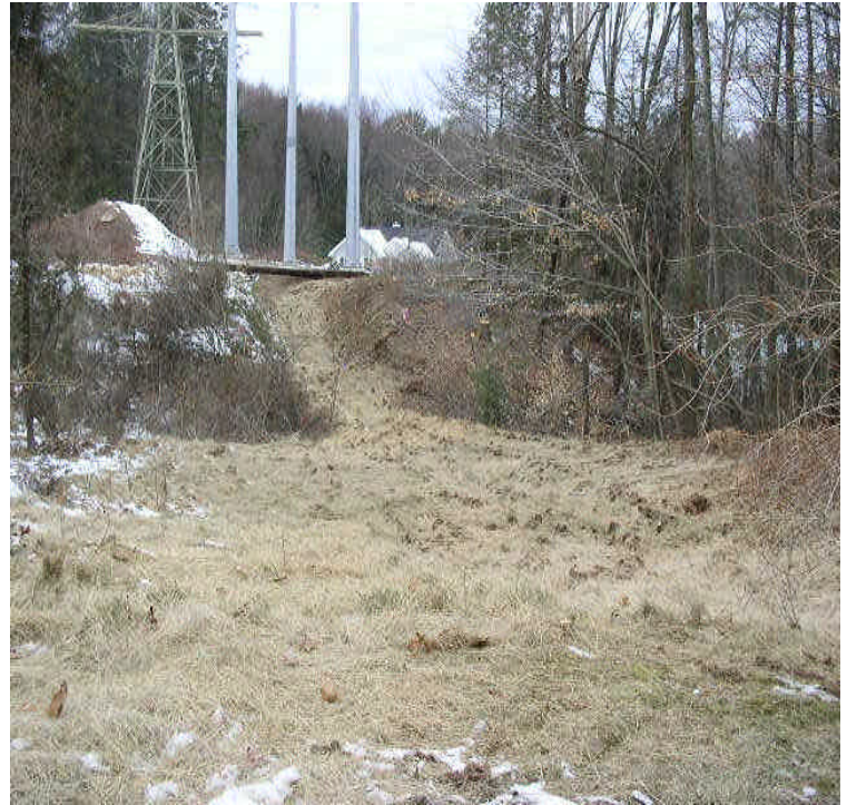
Old Farms Rd: View of the recently cleared wetland crossing. Mulch and seed were used for stabilization
