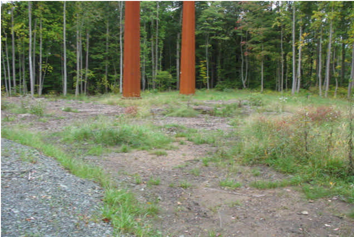
Vegetative cover is still sparse at the pad/angle structure. The area remains stable with thick wood chips but vegetation will not be able to establish fully. The contractor plans to remove the chips and seed the area when feasible.
