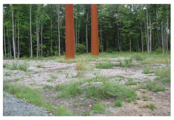
Vegetative cover is still sparse at the pad/angle structure. The area remains stable with thick wood chips but vegetation will not be able to establish fully. The contractor plans to remove the chips and seed the area when feasible.
