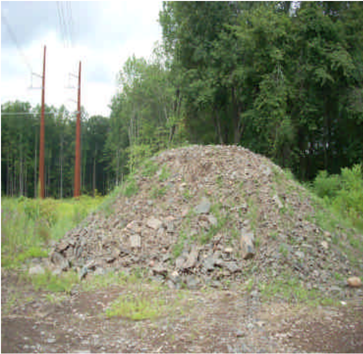
View of the stone/soil stockpile remaining in the contractor yard. Controls are in place but the pile is located just upgradient from wetlands and should be relocated.
