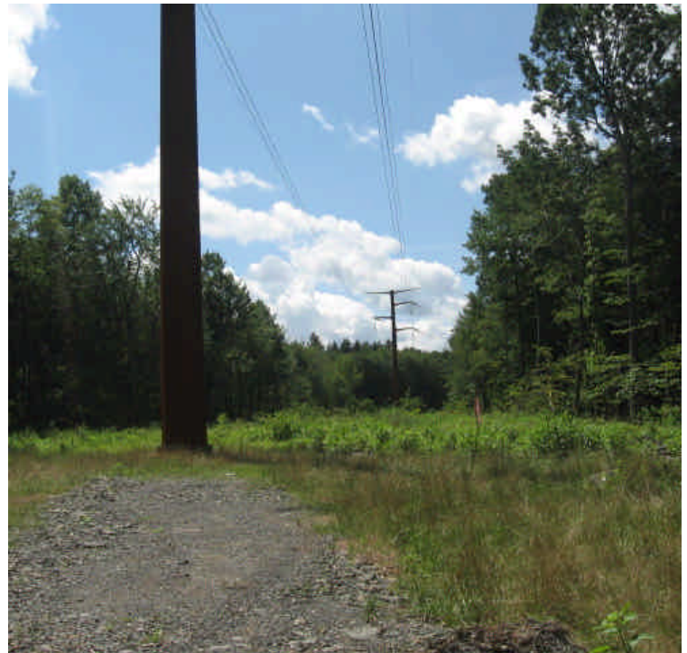
View of the ROW and wetland crossing looking towards Little Lane. The area has good vegetative cover, consisting of native wetland plant species.
