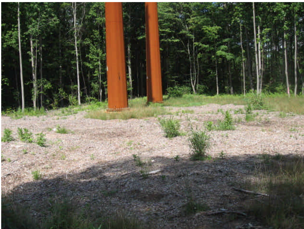
View of the pad/angle structure at the turn in the ROW off the receiving yard. The area remains stable with thick wood chips but vegetation will not be able to establish fully. The contractor plans to remove the chips and seed the area when feasible.
