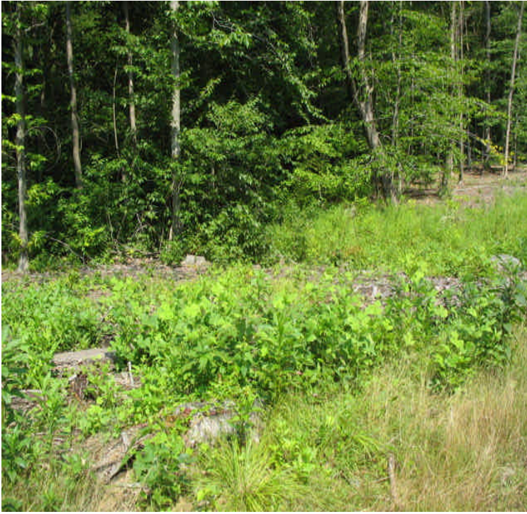
View of the turn in the ROW towards Little Lane off the Receiving yard. Silt fence was removed where adjacent areas are stable. A line of fence remains near the pad with thick wood chips.
