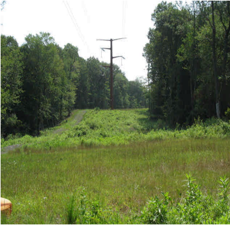
Vegetative cover noted along the ROW coming from the direction of Black Walnut Drive.
