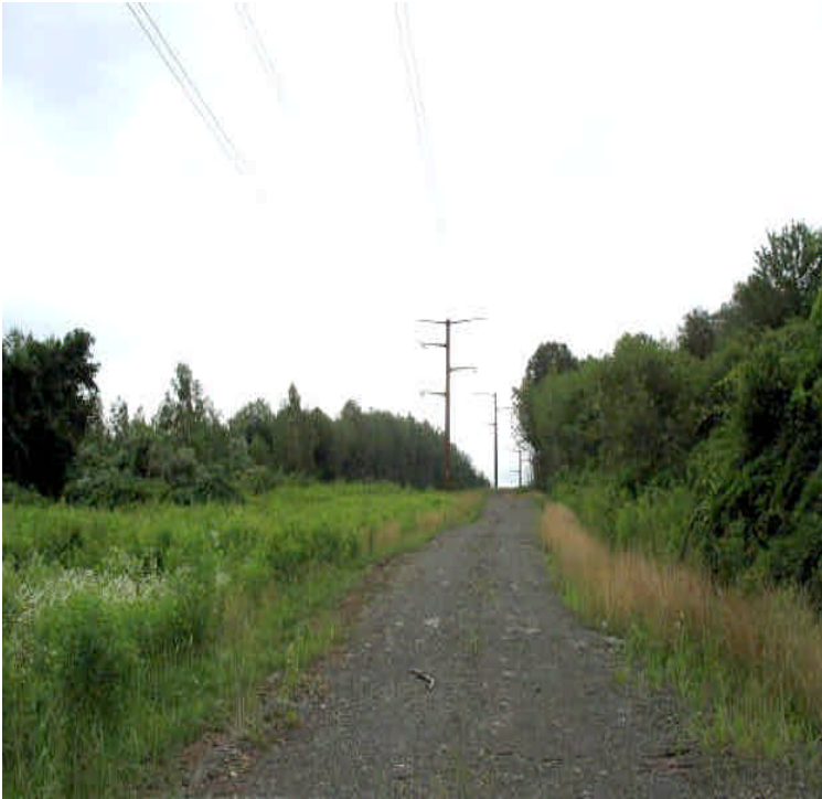
Grass growth noted along the ROW across from the receiving yard.
