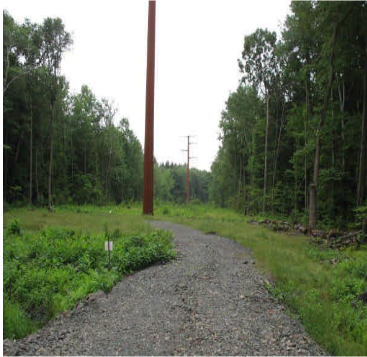
End of the access road from the receiving yard looking south.
