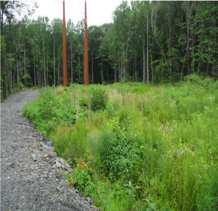
Wetland crossing at the edge of the receiving yard is stable.
