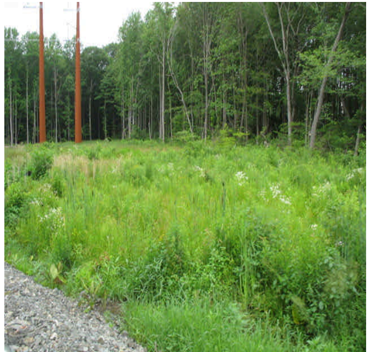
Wetland crossing at the edge of the receiving yard is stable with good vegetative cover.
