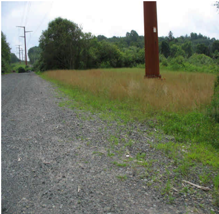
Grass growth noted at the pad site within the receiving yard.
