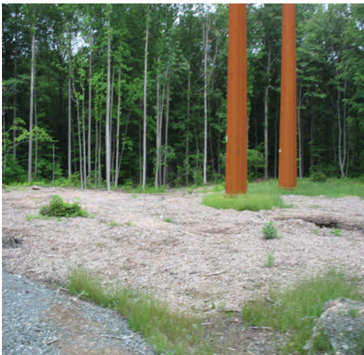
The pad at the turn towards Little Lane off the Receiving Yard has thick mulch/chips that are inhibiting vegetative growth.
