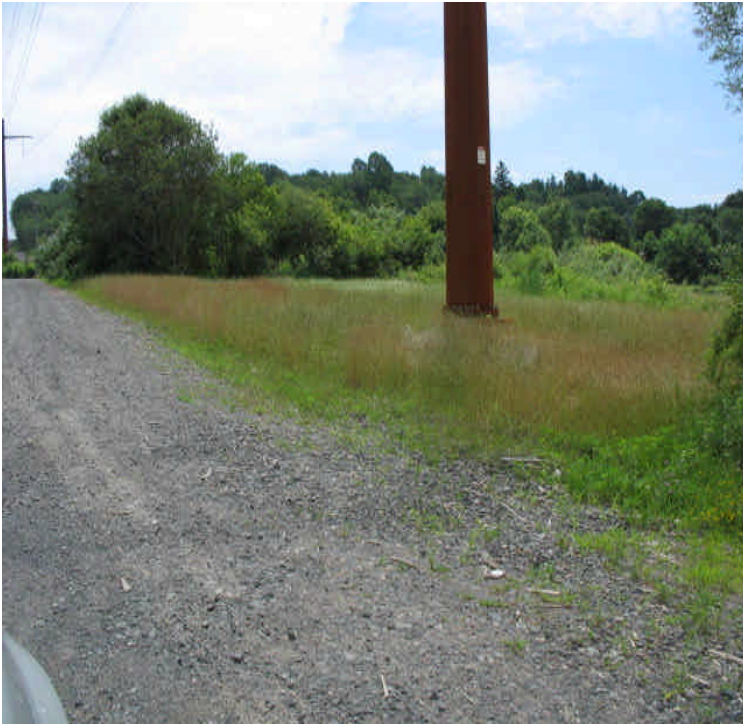
Grass growth noted at the pad site within the receiving yard.
