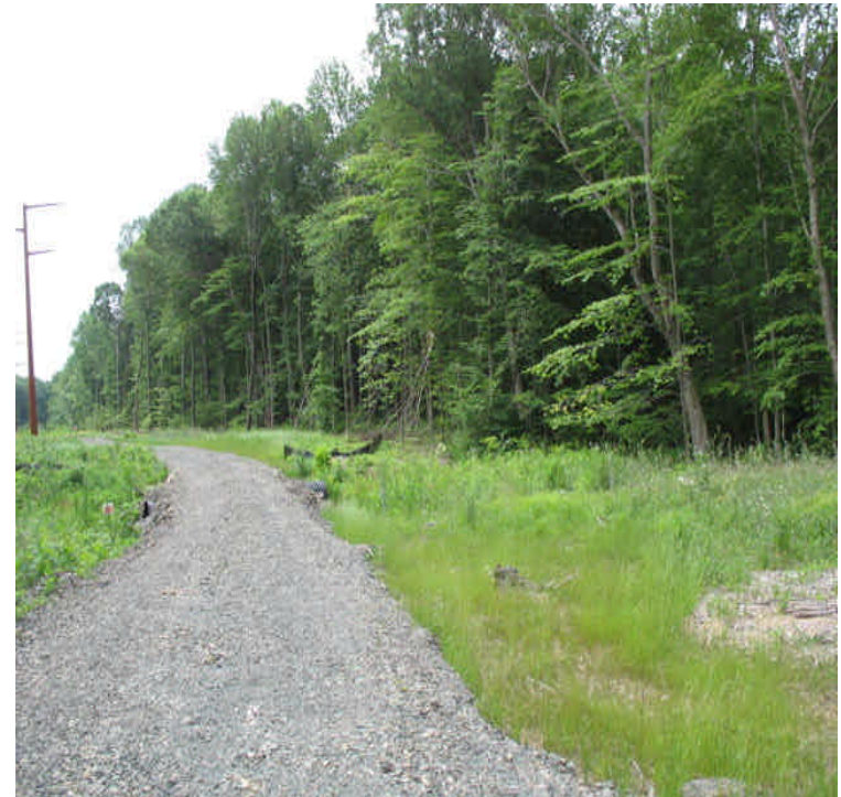
The majority of the ROW is stable with vegetation.
