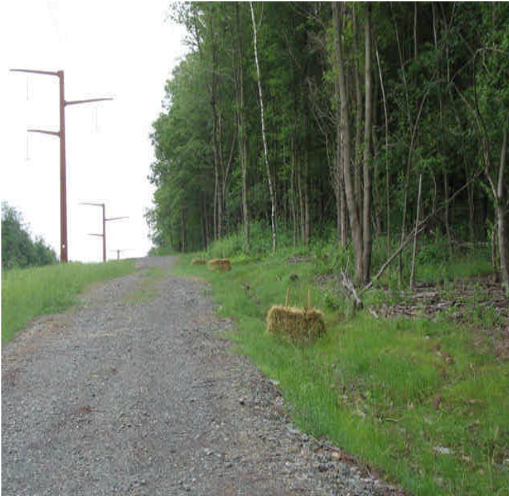
Grass growth noted at previously seeded areas along the access road across from the receiving yard.
