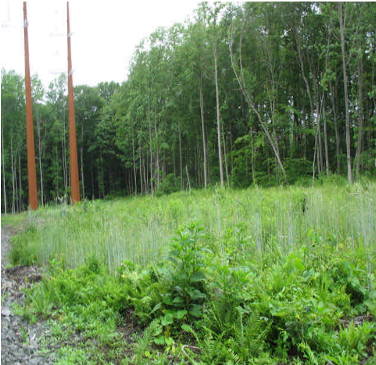
Previously seeded areas along the ROW have good vegetative cover. Remove any remaining silt fence where applicable.
