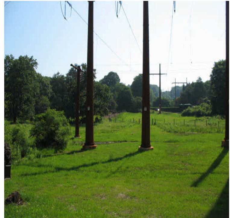
Final stabilization complete at the 1A & 1B connection off Little Lane. Areas have over 75% vegetative cover.
