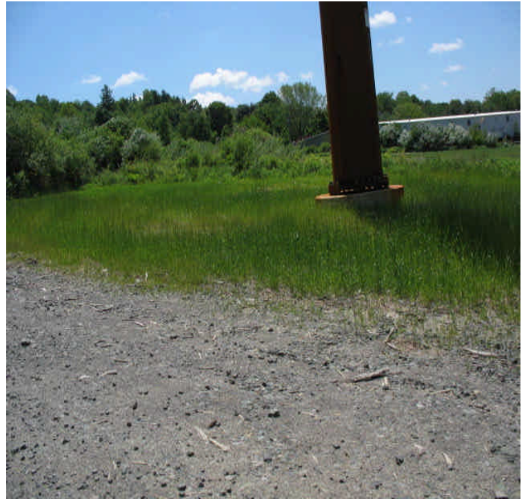
Grass is established at the structure within the receiving yard.
