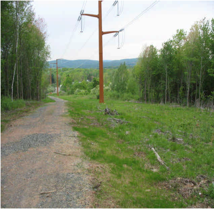
Grass and vegetative growth noted along the slopes east of the contractor yard to Black Walnut Drive.
