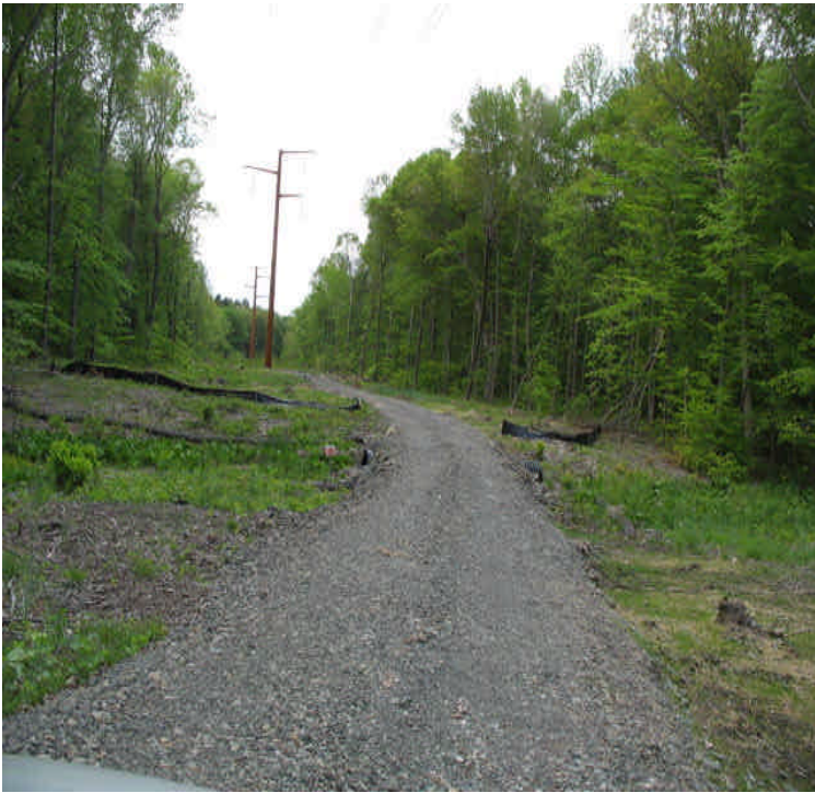
View of permanent wetland crossings looking north toward Little Ln.
