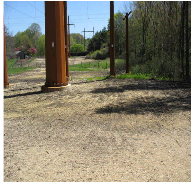
Timber mat removal and final grading from Rte 17 to Little Ln is complete. Monitor for final stabilization with vegetative cover.
