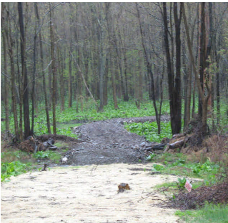
Water levels were higher at the channel bisected by the new access road. Either reduce the grade or install a culvert to maintain flow/hydrology in this area. Contractors will be evaluating this area but improvements will likely wait until a low flow period.
