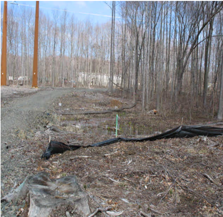
Wetland crossing and pad sites are awaiting reclamation within the watershed
