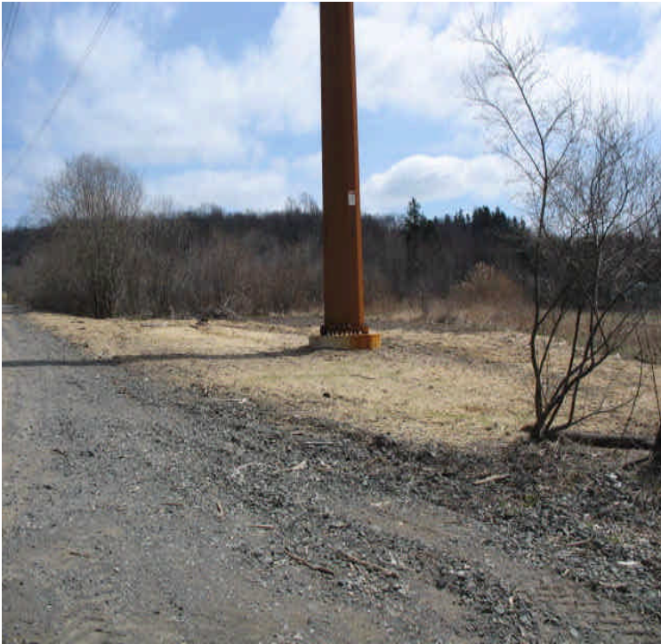
View of reclaimed pad within the receiving yard.
