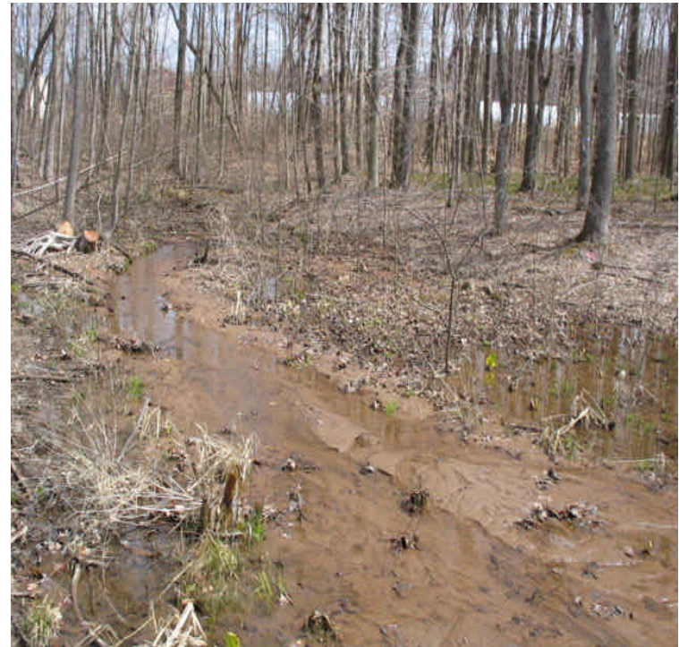
Controls remain in place at the access road stream crossing from the receiving yard. It appears that some sediment from the pond has settled accumulated within the wetlands. It is likely that sediment in the pond is due to the landowner and not project activities. However, consider carefully removing the sediment at this location.
