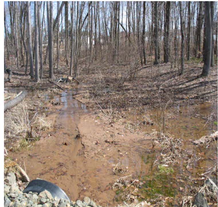
Controls remain in place at the access road stream crossing from the receiving yard. It appears that some sediment from the pond has settle accumulated within the wetlands. It is likely that sediment in the pon is due to the landowner and not project activities. However, consider carefully removing the sediment at this location.
