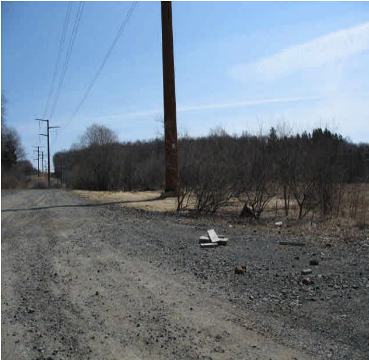
View of mulch and seed over the exposed area within the receiving yard.
