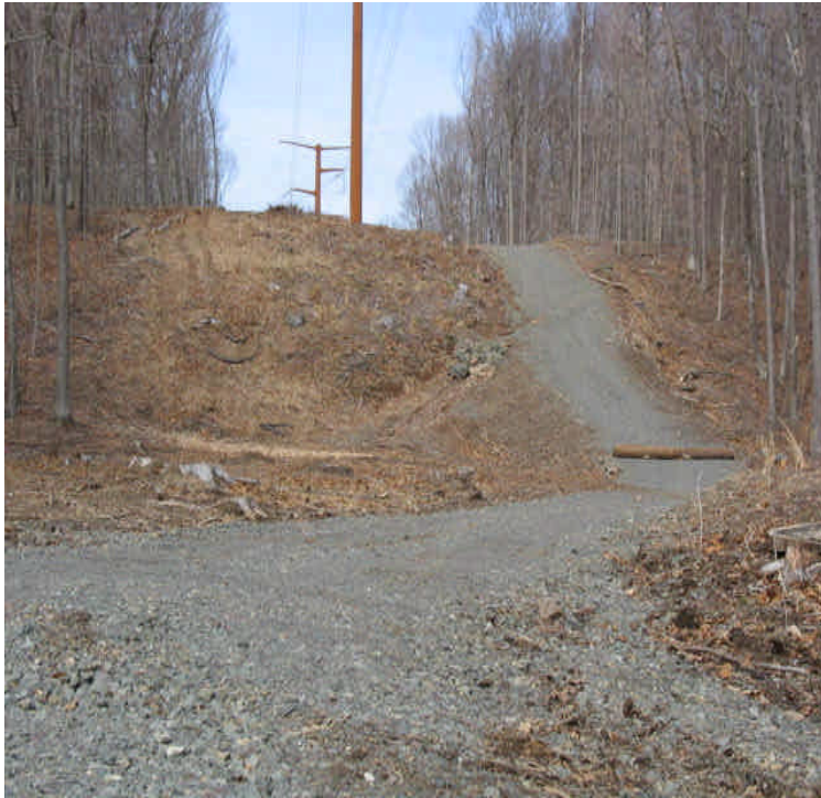
View of site entrance off Black Walnut Drive with water bar controls.
