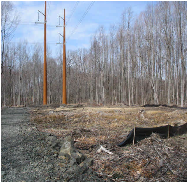
Hay and seed were applied over the reclaimed pull site. Silt fence remains in place adjacent to the wetland.
