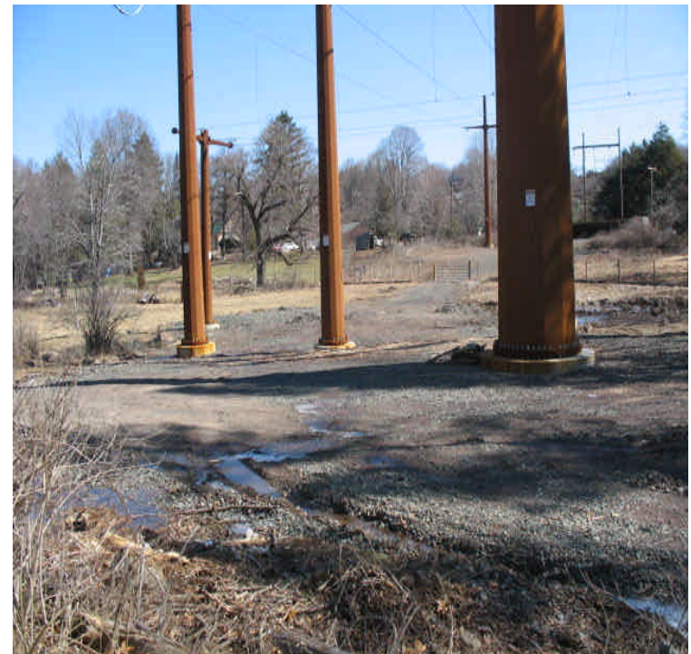
View of the 1A and 1B intersection off Little Lane. Controls are in place. Reclaim the pad sites when feasible.
