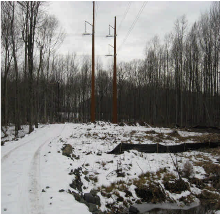
View of the exposed stockpiles. Topography here appears to reduce the potential of run-off to wetlands.
