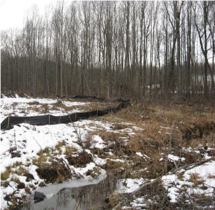
Controls remain around the old pull site. Stabilize/restore soils as soon as feasible.
