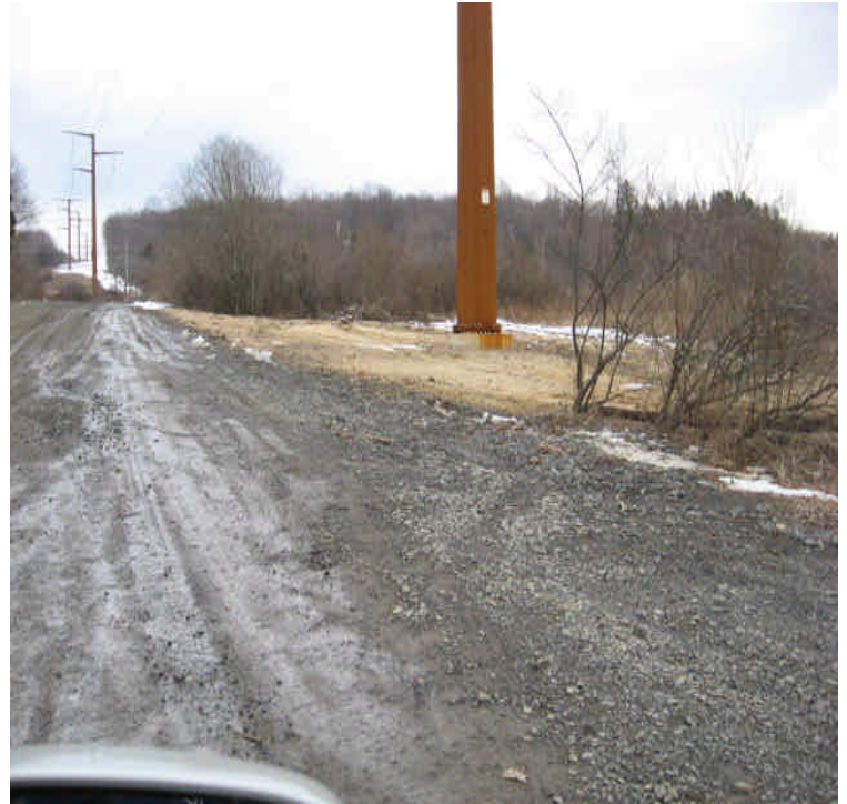
Exposed/reclaimed areas remain mulched and seeded west of Rte 17 in the receiving yard.
