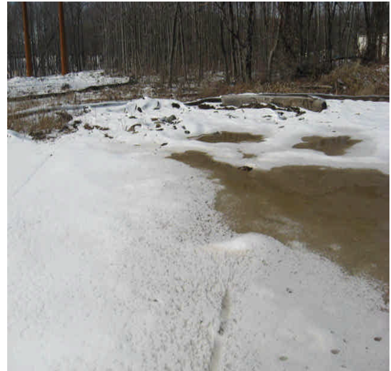
Turbid water is pooling at the edge of the receiving yard. However, it was observed filtering through controls before entering the wetland
