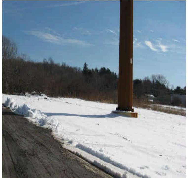
Prior to snow cover, exposed/reclaimed areas had been mulched and seeded west of Rte 17 in the receiving yard.
