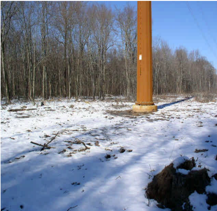
Timber mats have been removed from the Rte 17 access near Little Ln. Stabilization is needed when weather conditions permits.
