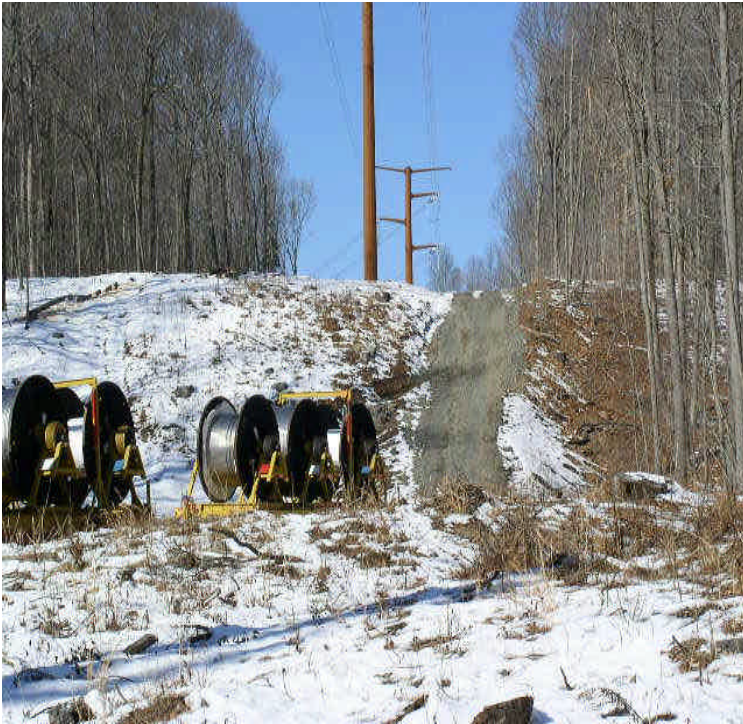
The slope off the Black Walnut Dr. entrance has a drainage ditch/water bar to divert run-off and an old wooden pole to prevent vehicles from driving over and damaging controls.
