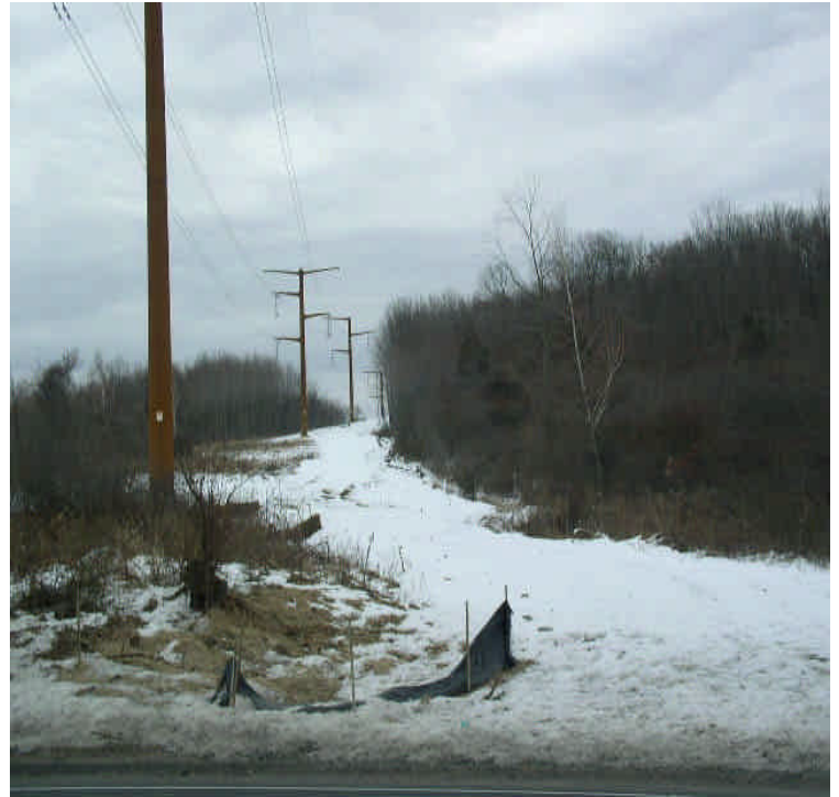
View from the Rt. 17 east entrance: Several areas have been reclaimed and mulch/seed are in place for temporary stabilization. Snow cover and freezing temperatures also help to stabilize.
