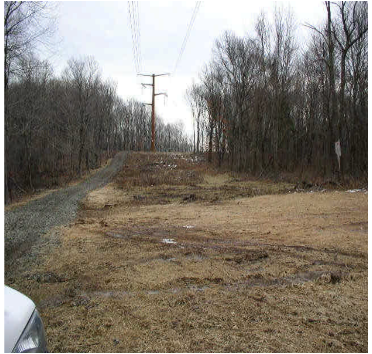
Recently reclaimed, seeded and mulched area off the Black Walnut Dr. entrance.
