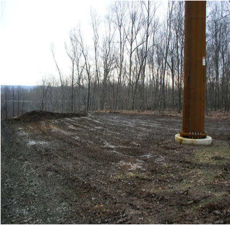
Recently reclaimed area near the Black Walnut Dr. entrance. Area should be temporarily stabilized with mulch for the winter.
