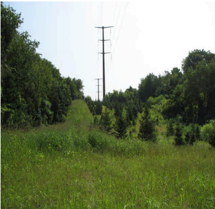
Powder Hill Rd: Vegetative growth/cover along the slope east off the roadway.
