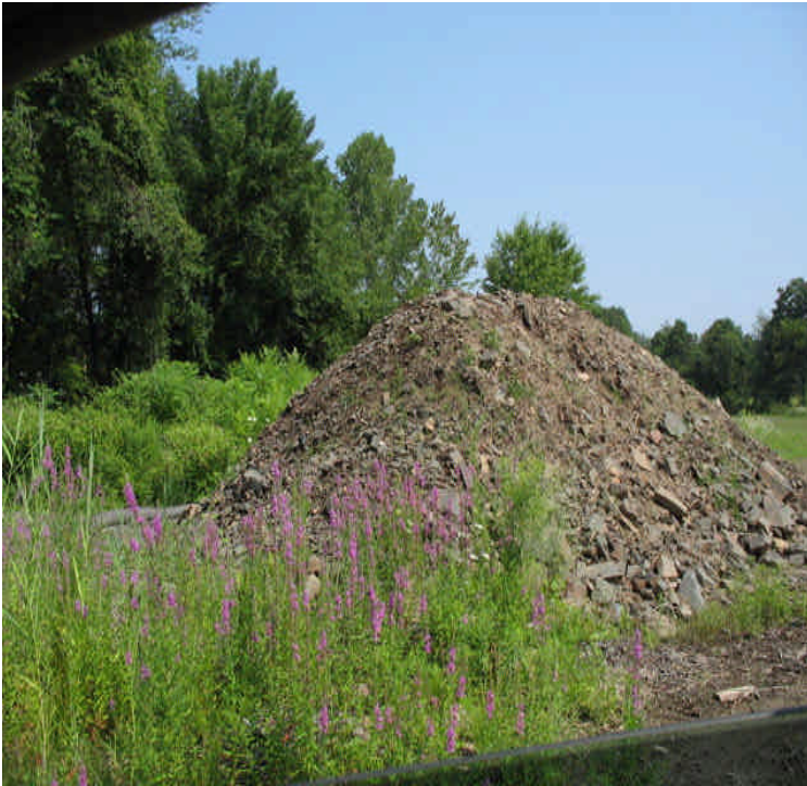
Contractor Yard: Stockpile located upgradient of the wetlands in the receiving yard. A filter sock is in place at the base of the pile.
