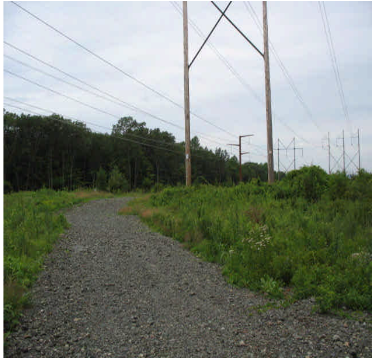
Bartholomew Rd: View of vegetative growth/cover west of the roadway.
