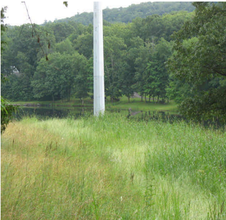
Fleming Rd: Vegetative growth/cover along the slope upgradient of the pond.
