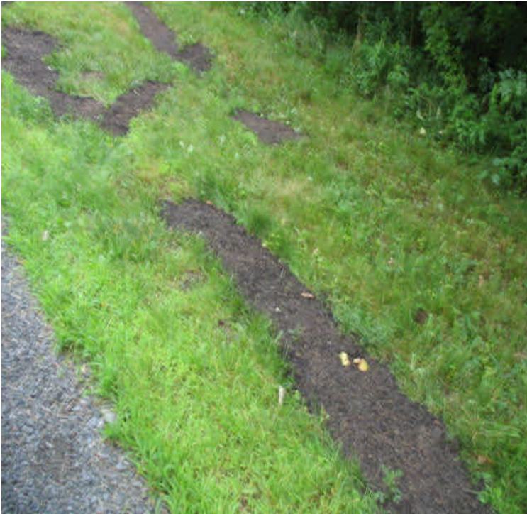
Rte 157: Small ruts along a private driveway east of Rte. 157 were filled in with topsoil and seeded.
