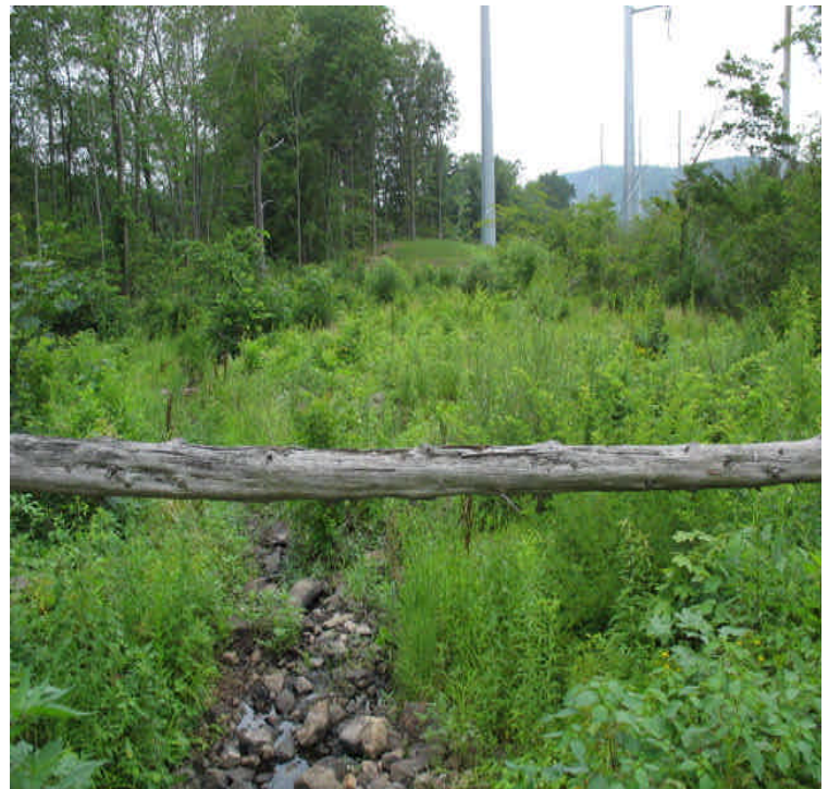
North of High Hill Rd: View of vegetative growth along the stream channel.
