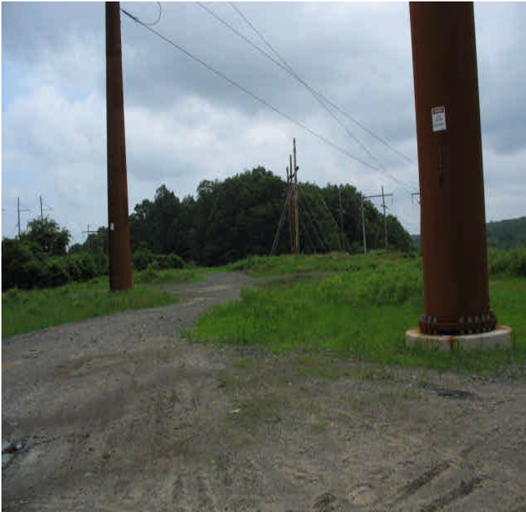
Oxbow Jct: View of vegetative growth/cover at Oxbow.
