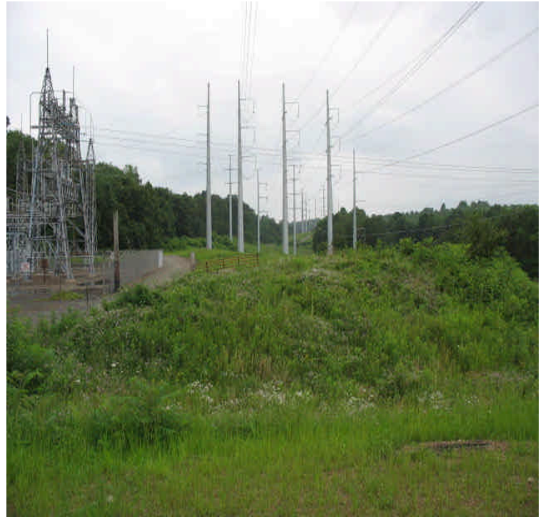
E. Meriden SS: View of vegetative growth adjacent to the switching station
