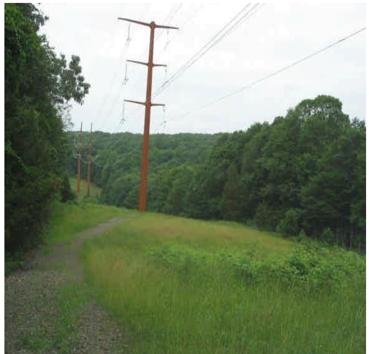
Arbutus St: Top of the slope looking toward Ball Brook and the last structure off Black Walnut Dr. Good grass cover was noted.
