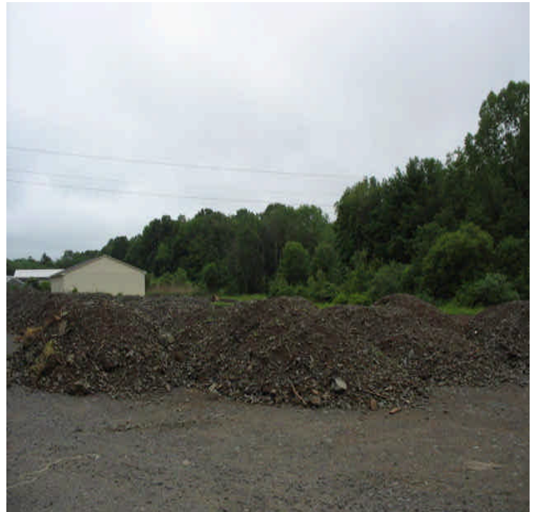
Contractor Yard: Remaining additional soil stockpiles from several sites should be temporarily stabilized or removed.
