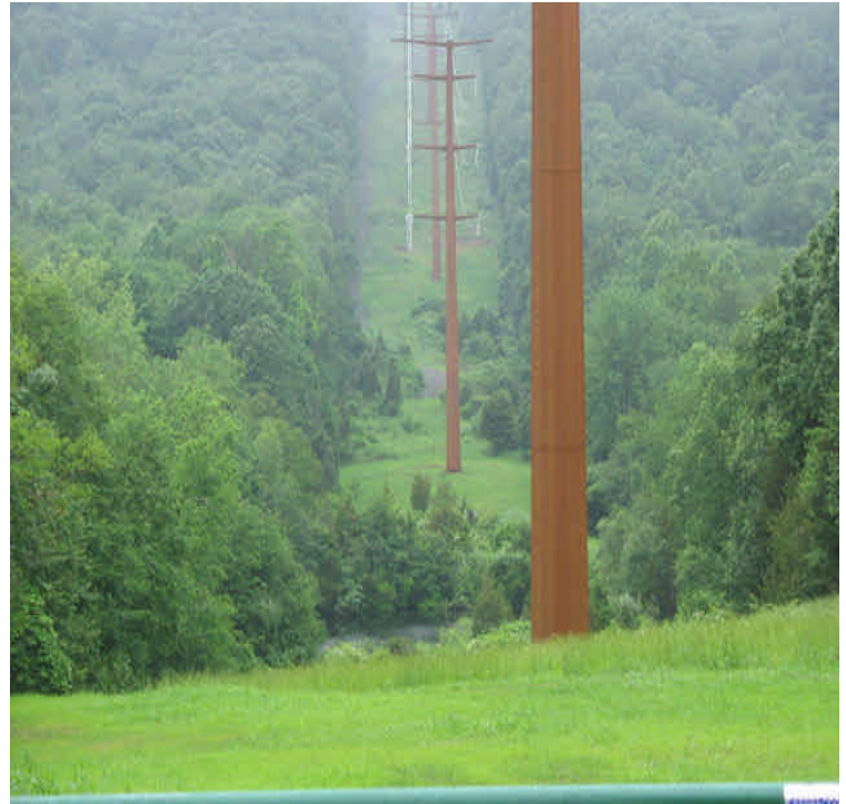
Powder Hill Rd: Final restoration complete. Grass growth noted along the slopes and the ROW is in good shape.
