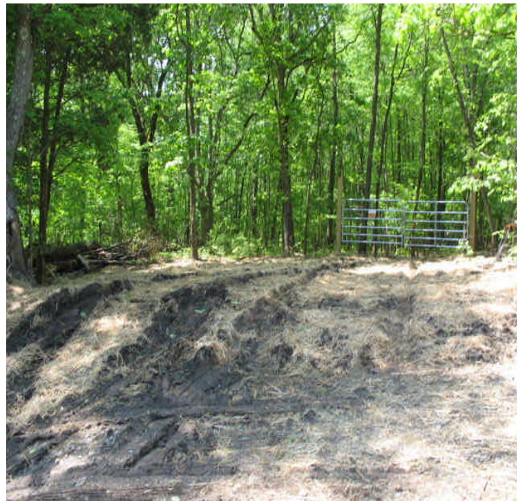
Shunpike Rd East: Final restoration complete off Shunpike Rd. It appears other vehicles are tracking through this area.
