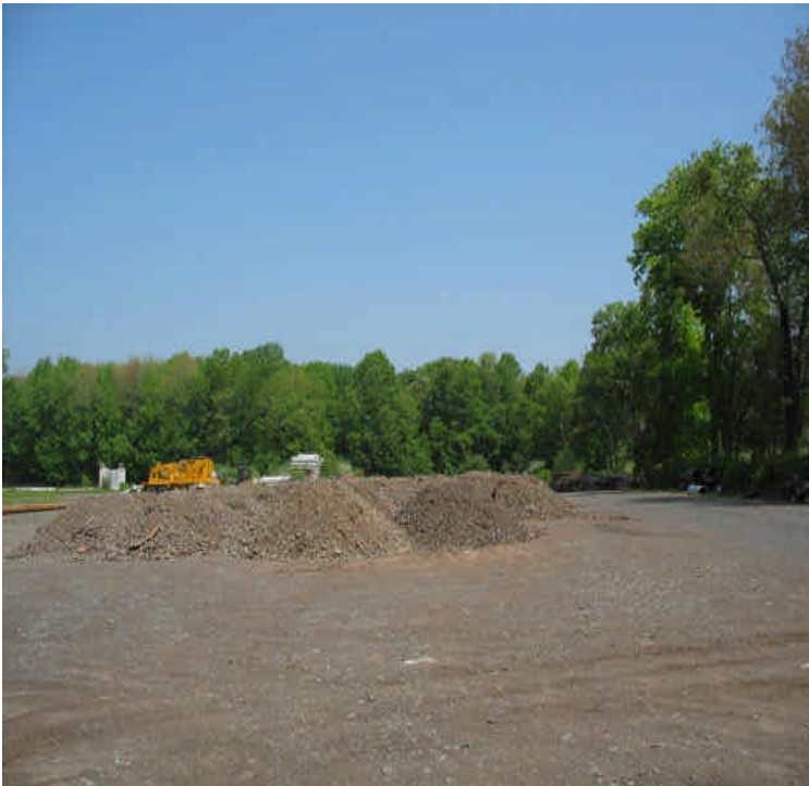
Contractor Yard: Stockpiling soils from restoration at Scovill SS to Chestnut Jct. Remove or stabilize as feasible.
