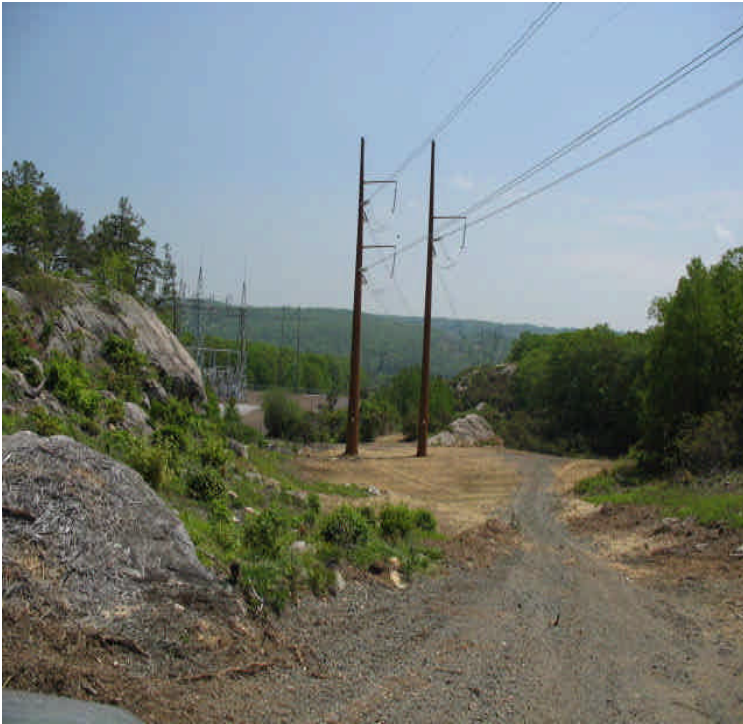
West of Scovill SS: Final grading and reclamation complete.
