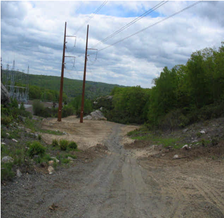
West of Scovill SS: Final grading and reclamation underway.
