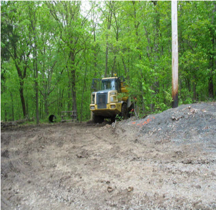
Shumpike Rd. West: Final grading and restoration measures underway.
