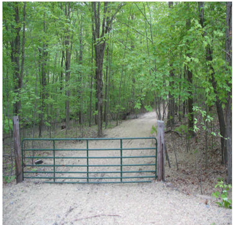
Shumpike Rd East: Final restoration complete from the eastern access to Rte 9
