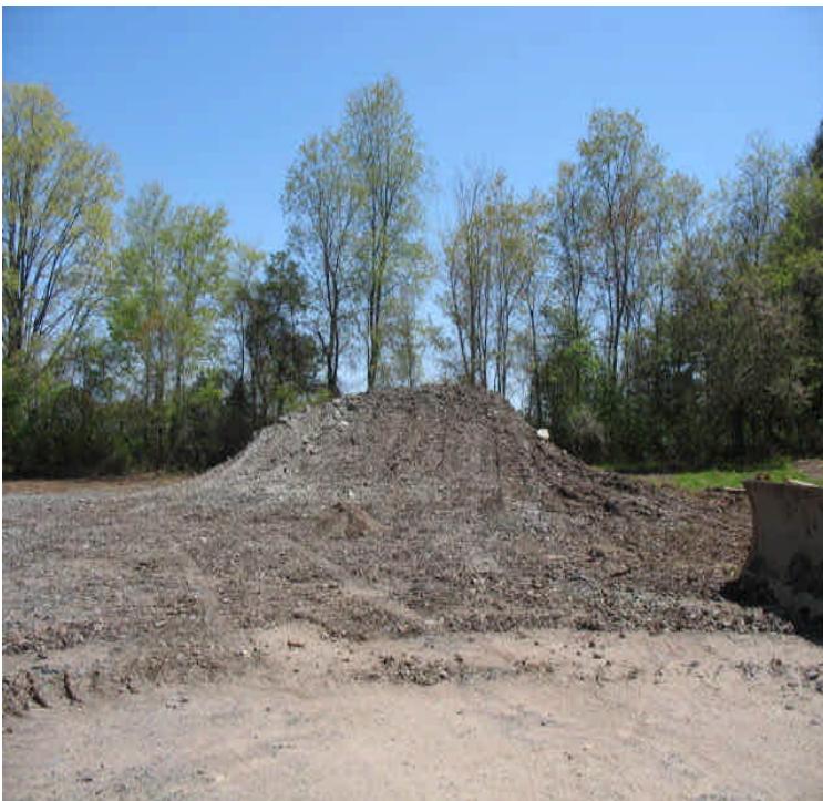
Contractor Yard: Stone and soil stockpiles from Black Walnut Dr. were stockpiled at the edge of the field staging area. Controls or removal are needed.
