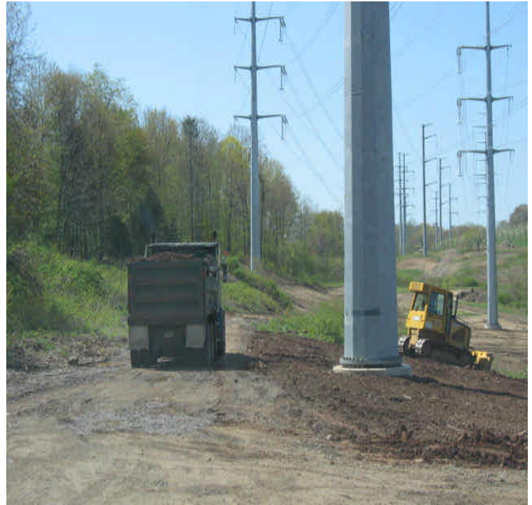
E. Meriden SS (south): Final grading and soil/stone removal is underway.
