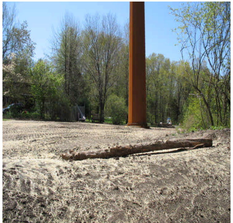
Little Lane: Final grading and stabilization are complete.
