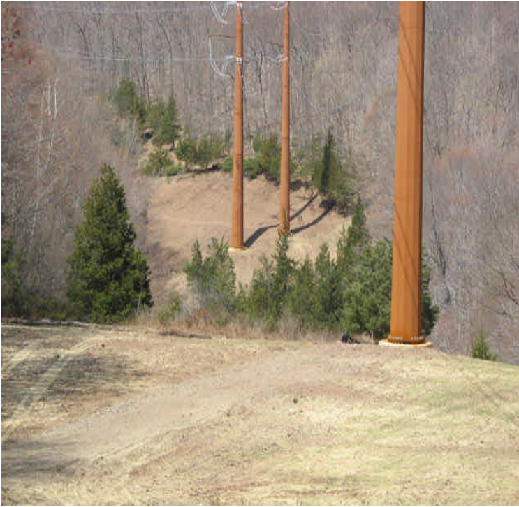
Arbutus St to Black Walnut Dr: Final mulch and seeding complete at Arbutus. However, additional mulch and seed needed on exposed slope off Black Walnut.
