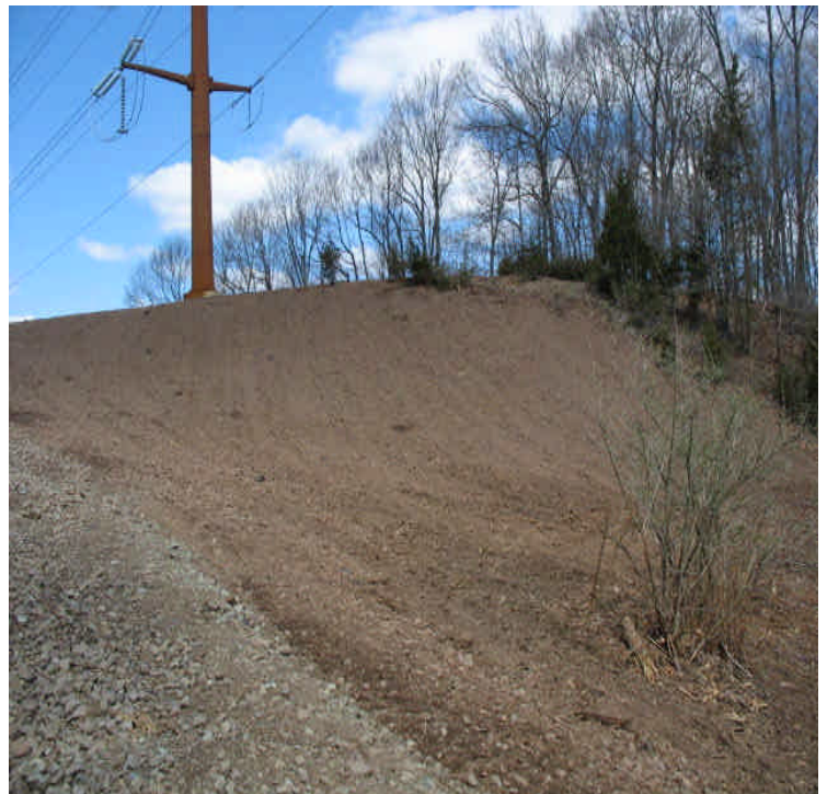
Arbutus St: Restoration almost complete west off the roadway. Final grading is complete, however hay/seed and controls are needed until the area is stable.
