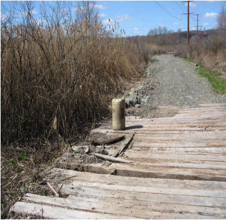
Durham Rd: It appears a non-project related container was dumped on the mats at the edge of the wetland. The container was ½ filled with a liquid that appears to be oil.
