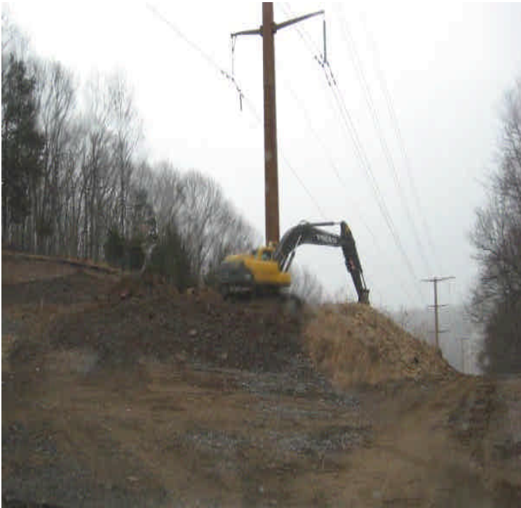
Arbutus St: Grading and pad restoration underway.
