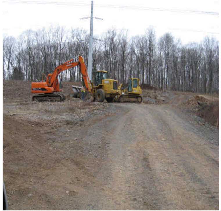
North of BSS: Reclamation continues moving north from BSS.
