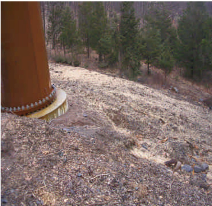
Black Walnut Dr: Final reclamation almost complete upgradient from Ball Brook. Continue to monitor this slope due to high potential for erosion.
