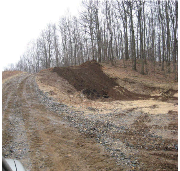
Arbutus St: Another view of the grading and restoration activities.
