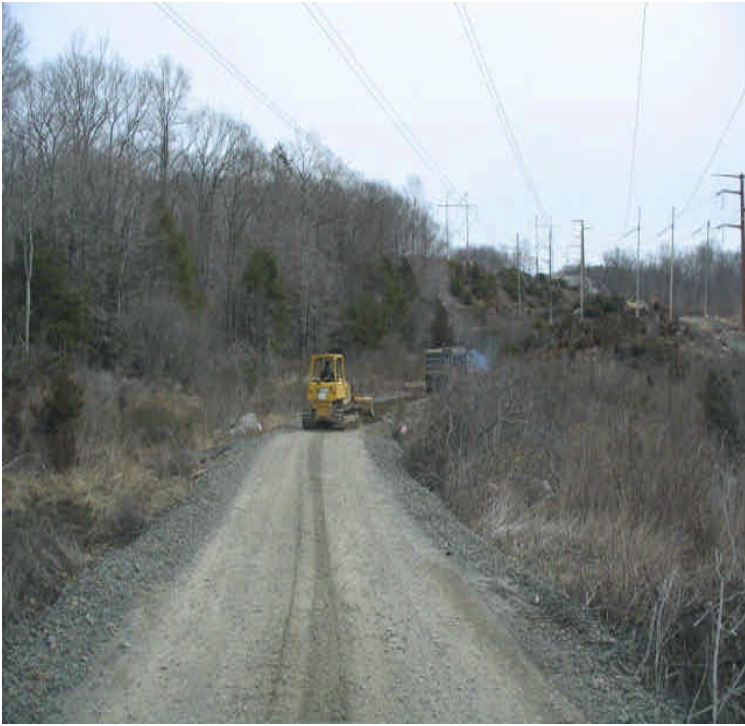
West of Scovill SS: Access road work is underway.
