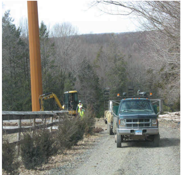
Foot Hills Rd: Crews were reclaiming pads and stabilizing soils.
