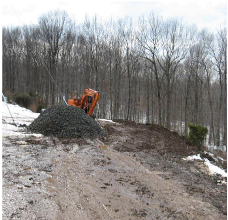
East Mount Rd: Access road and pad installation underway.
