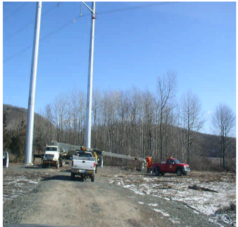
South of E. Main St: Line work underway adjacent to wetlands.
