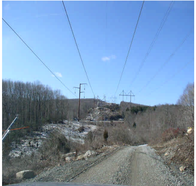
Route 9 Crossing: Line work was underway.
