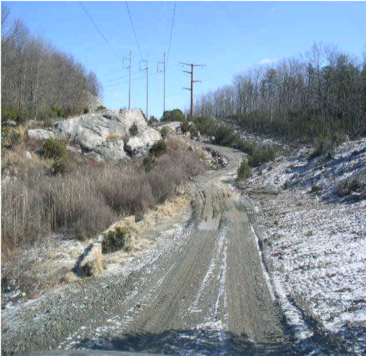
West of Scovill SS: Haybales installed to stop run-off to wetland #5.
