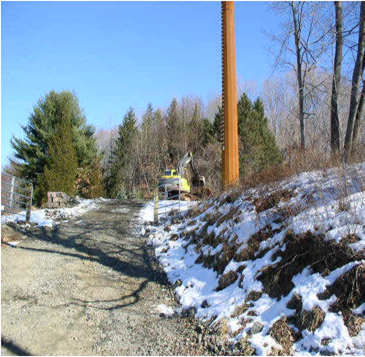
Foot Hills Rd: Minor grading and pad work was underway.
