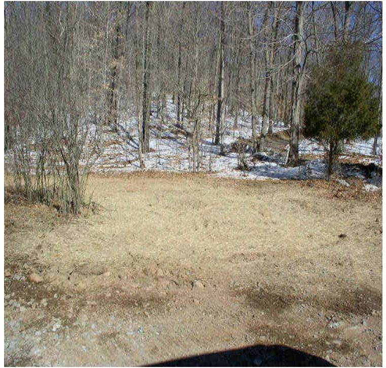
Johnson Ln: A small stockpile was removed and the area was mulched and seeded
