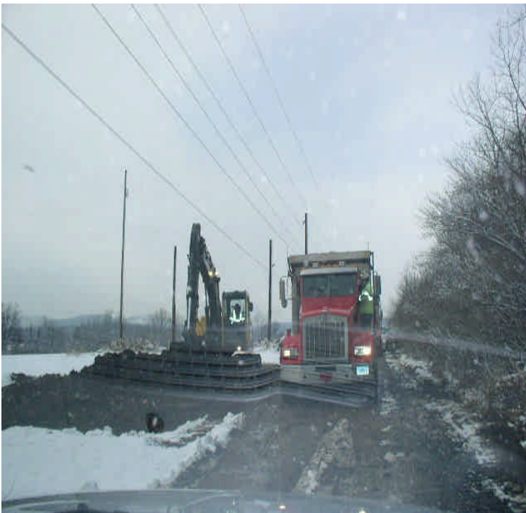
Little Lane: Stockpile removal underway. Line pulling activities were also occurring.
