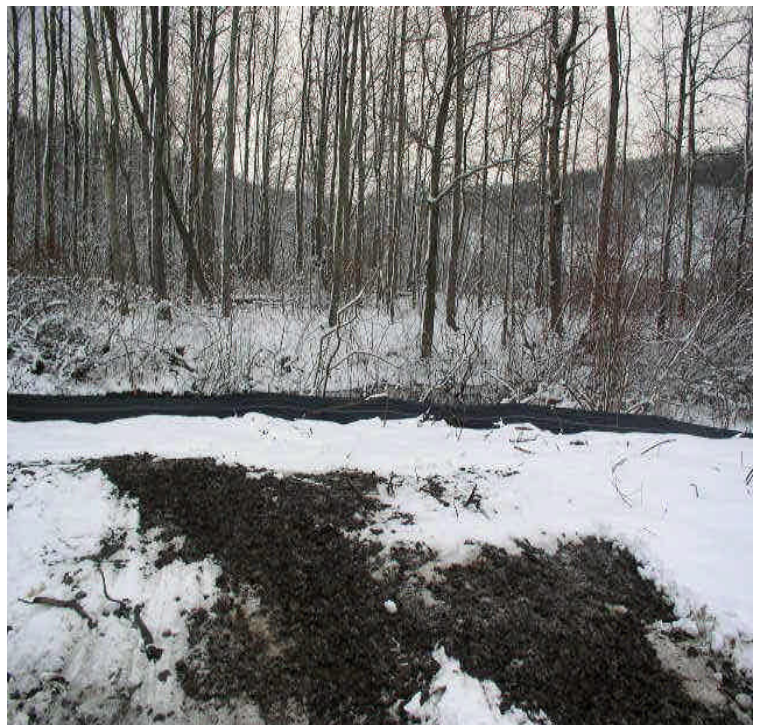
South of East Main Street: Snow and associated sediment have been removed from the wetlands and controls have been installed.
