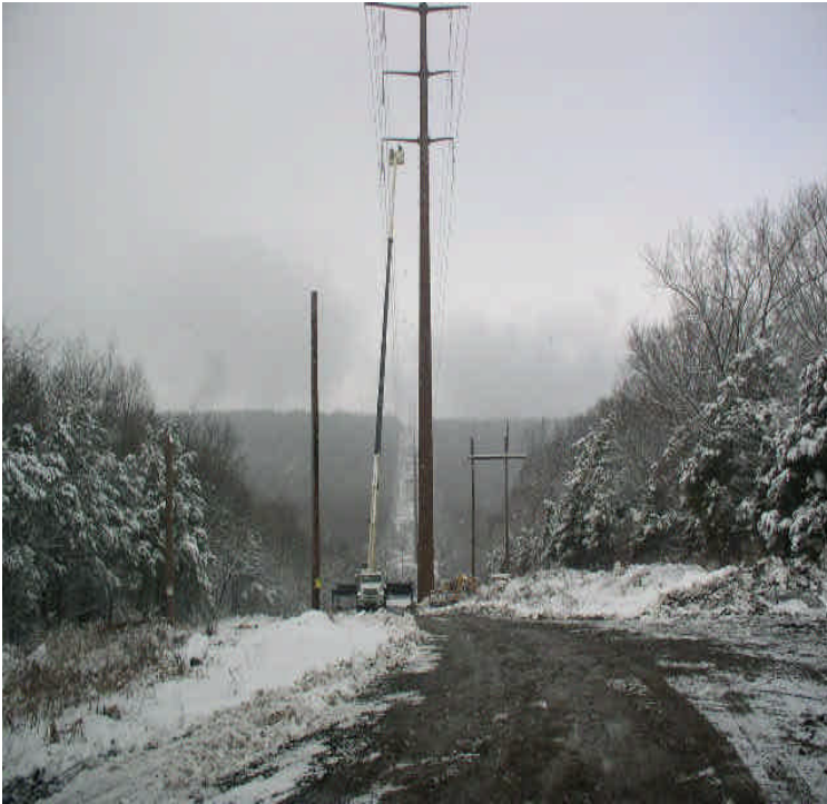
Powder Hill Rd: Line work underway between here and Little Lane.
