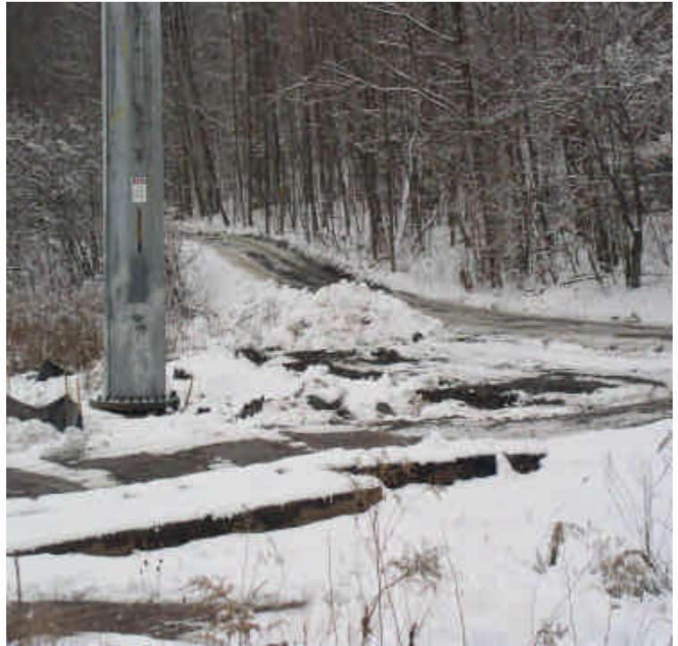
High Hill Rd: Provide controls in order to reduce sediment tracking on the timber mats as needed. Controls are still needed upgradient from wetlands in this section.
