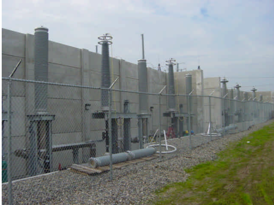
Tie-in work continues inside the Norwalk substation.
