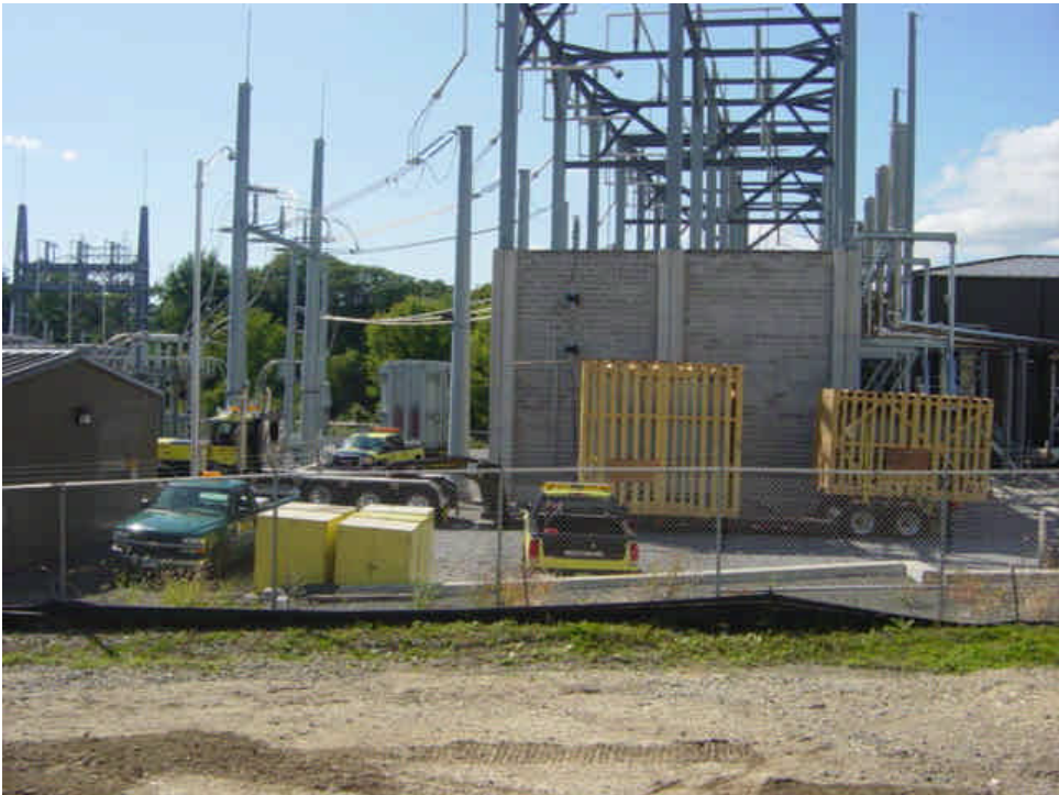
New electrical equipment was delivered to the Norwalk Substation.
