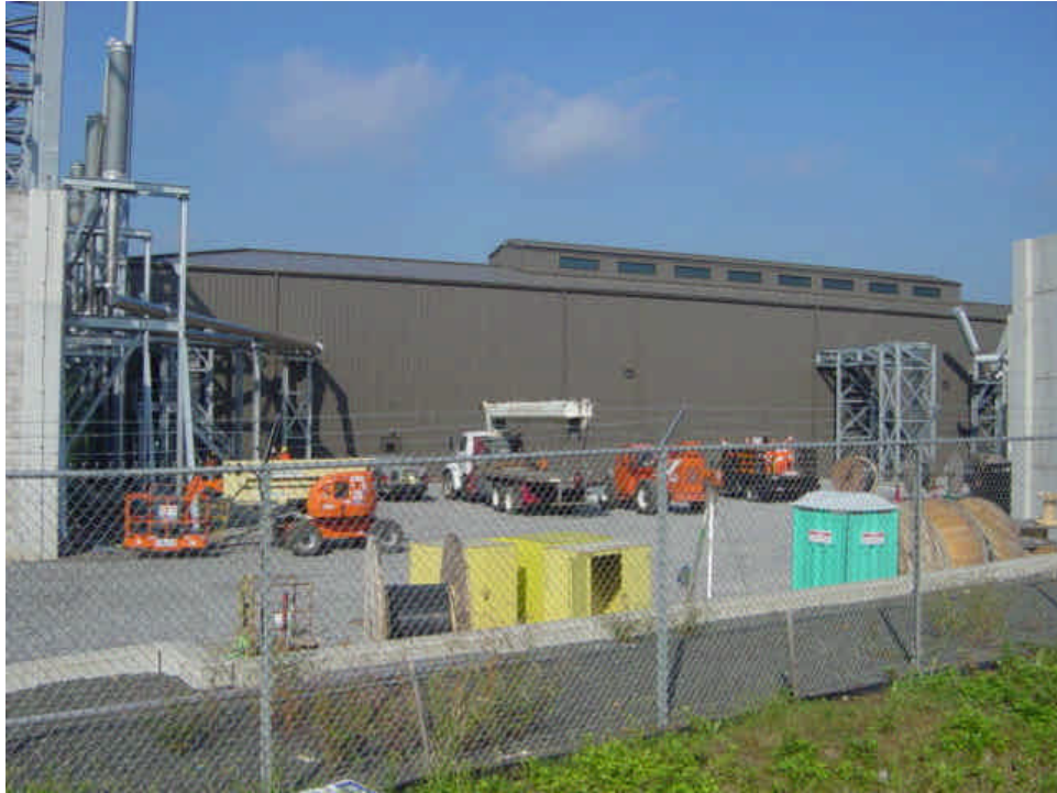
Electrical tie-in work continues inside the substation perimeter.
