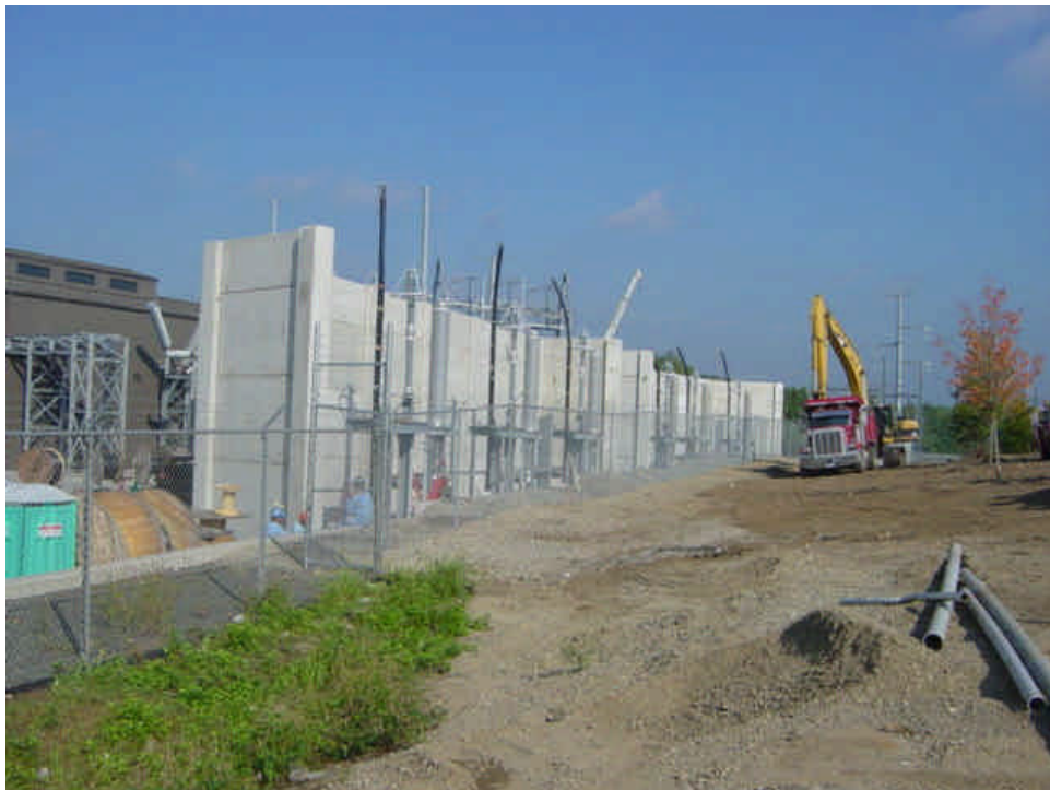
Electrical connection and tie-in work continues inside the substation perimeter.
