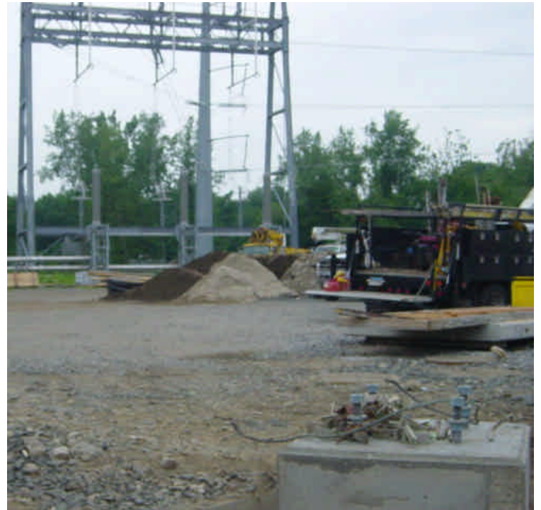
Stockpiled material was appropriately contained with silt fence.
