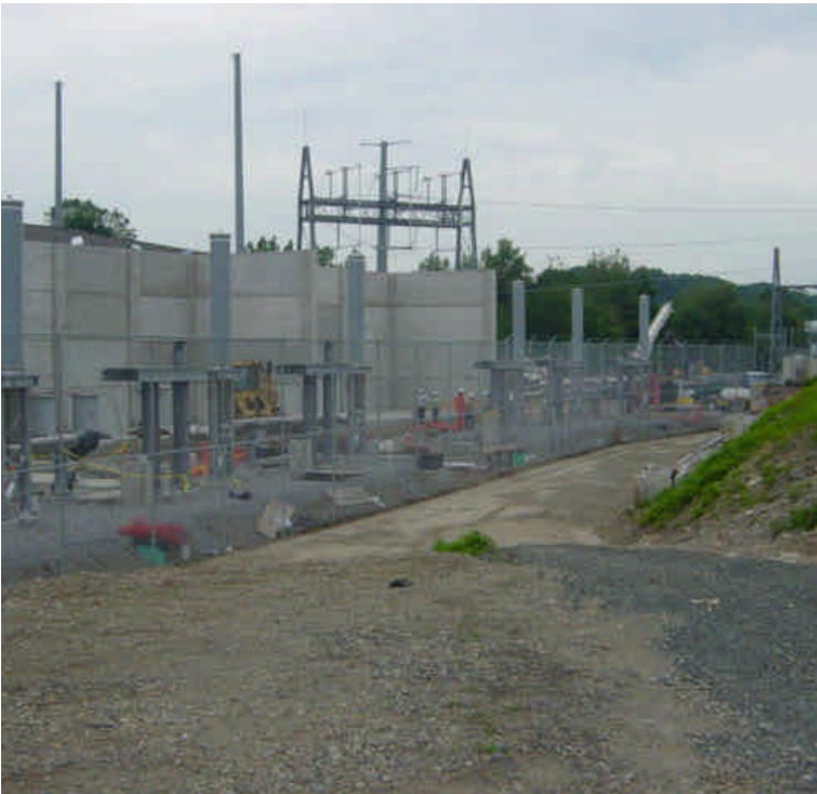
Additional concrete foundations have been placed within the substation.
