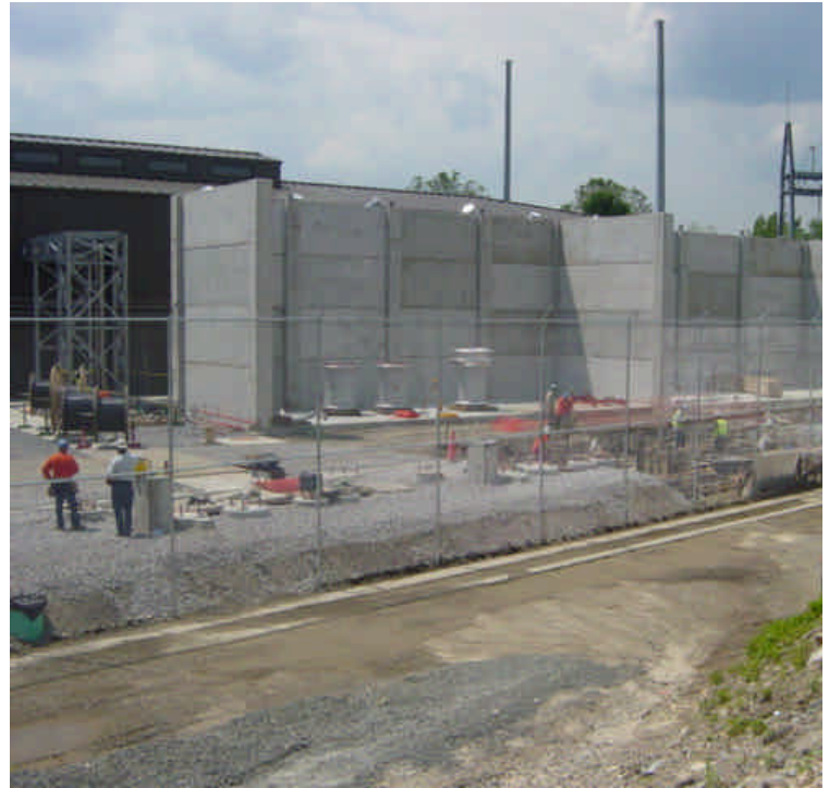
Crews were on-site preparing to pull cable and place additional equipment.
