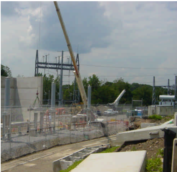
Additional electrical equipment was being placed inside the substation.
