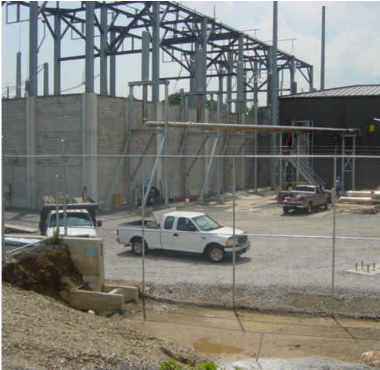
Electrical connection and tie-in work continues inside the substation.
