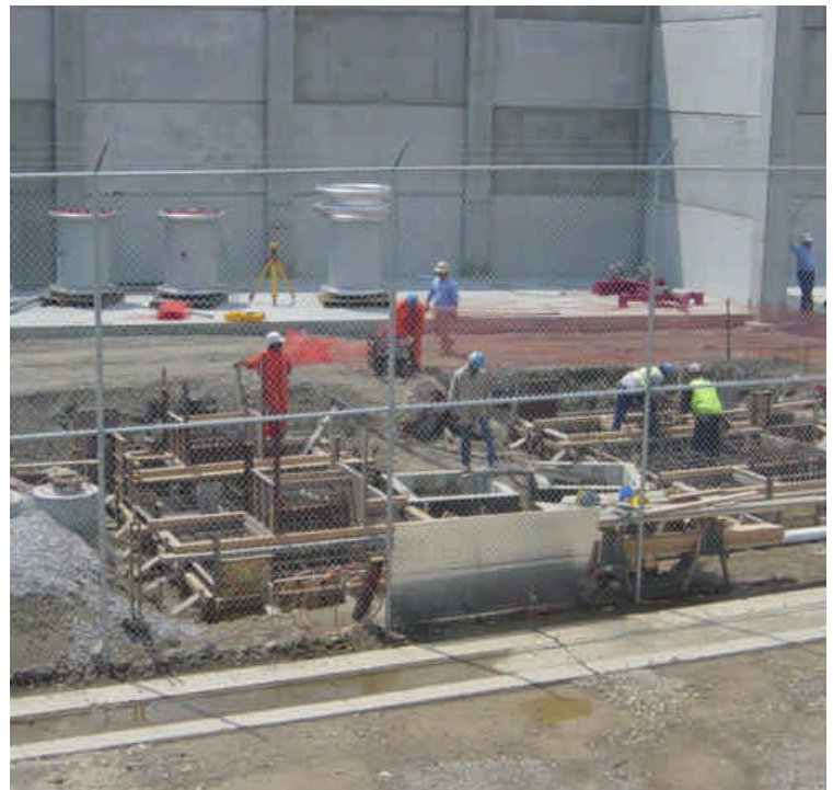
Crews were placing formwork in preparation for additional equipment foundations.
